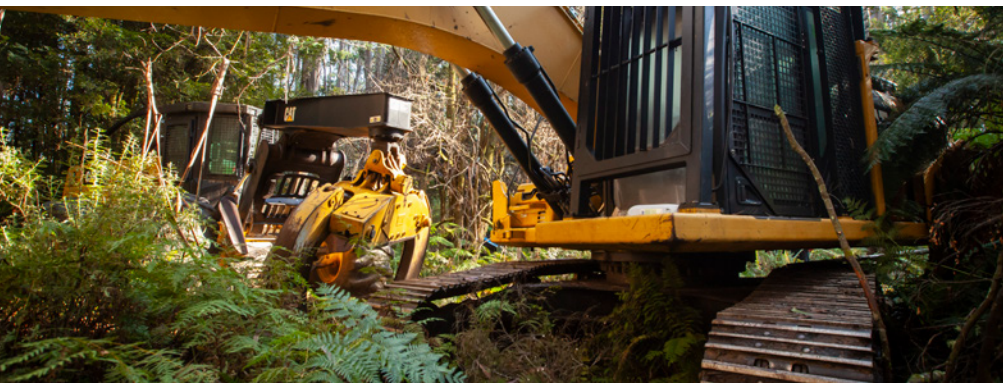
↑ Fire break works, Noojee
