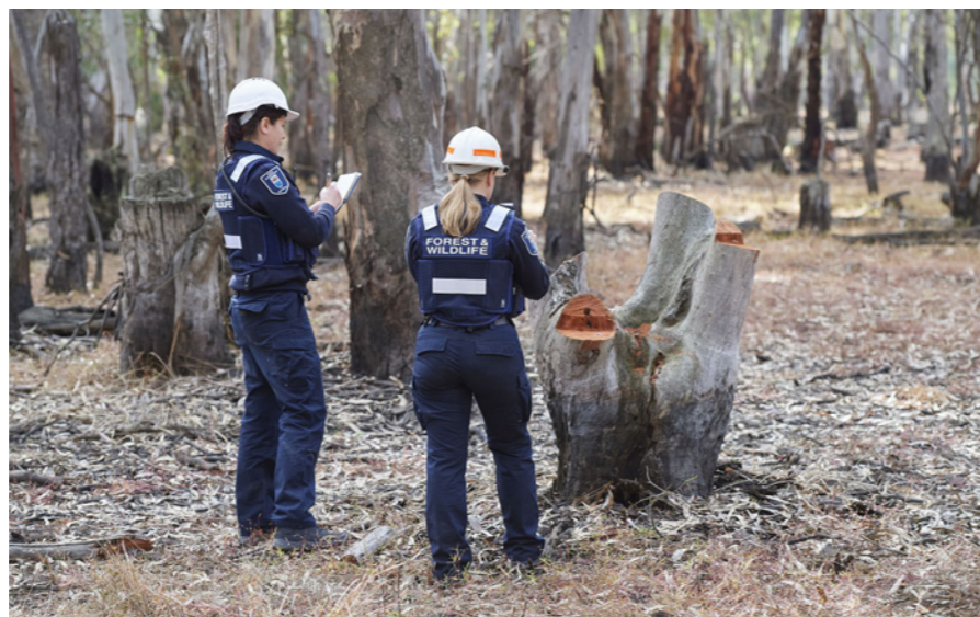
↑ Authorised Officers Jodie and Libby inspect damage from firewood thieves in the Gunbower State Forest CONSERVATION REGULATOR
