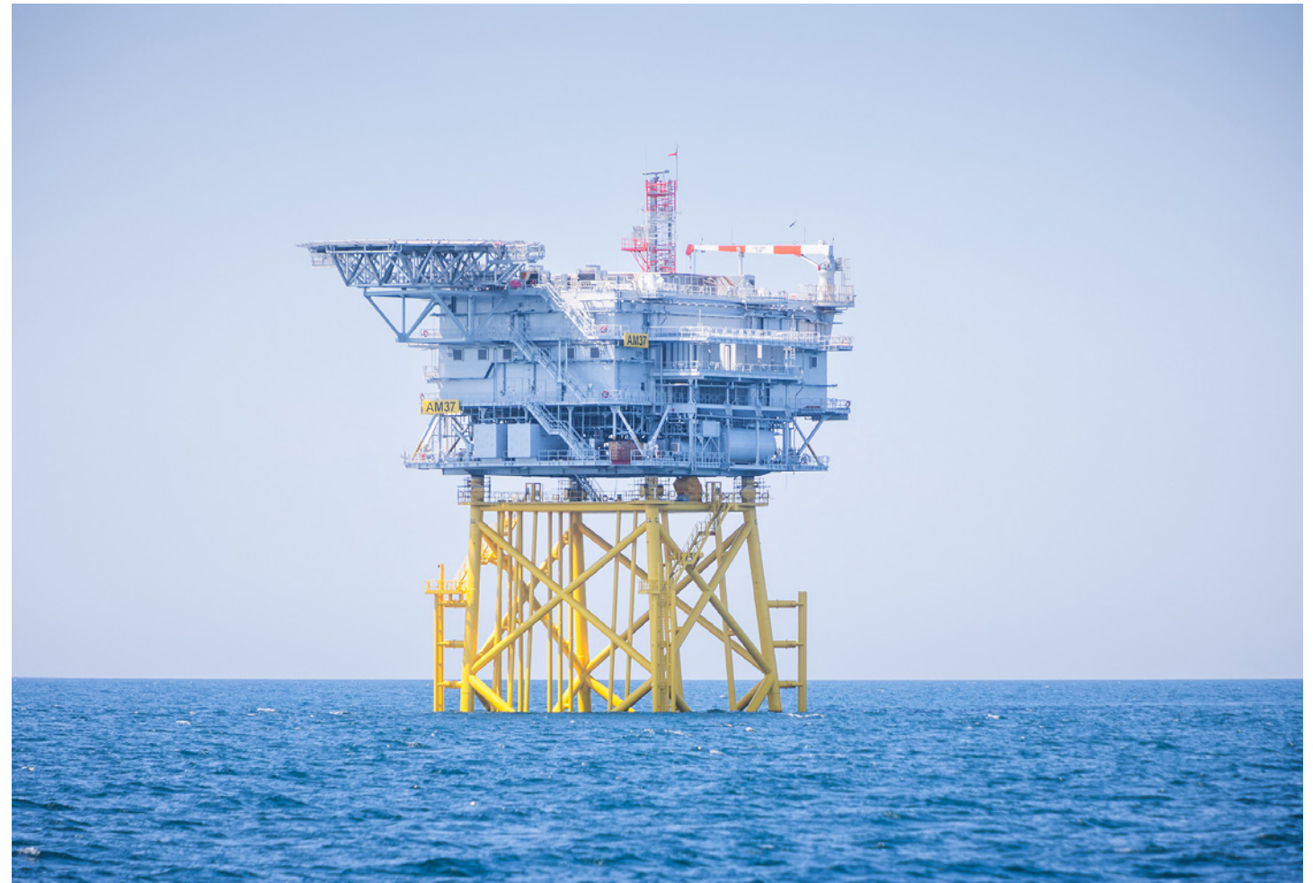
Vineyard Wind 1 offshore wind substation, United States. Avangrid
