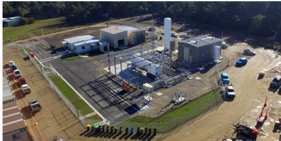
HESC Project site in Hastings. SOURCE: HESC
