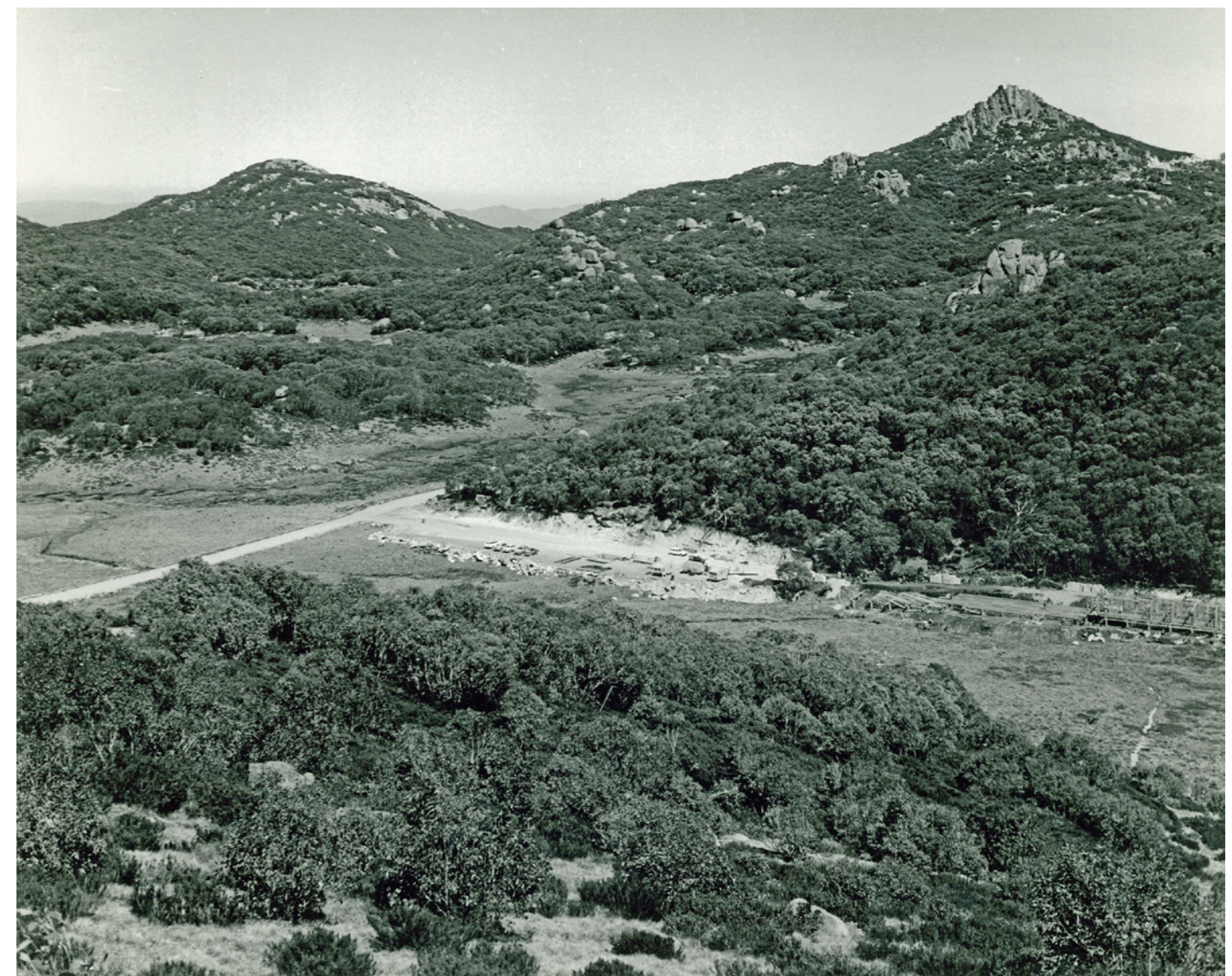
Tatra Inn under construction at Mt Buffalo National Park, early 1960s
