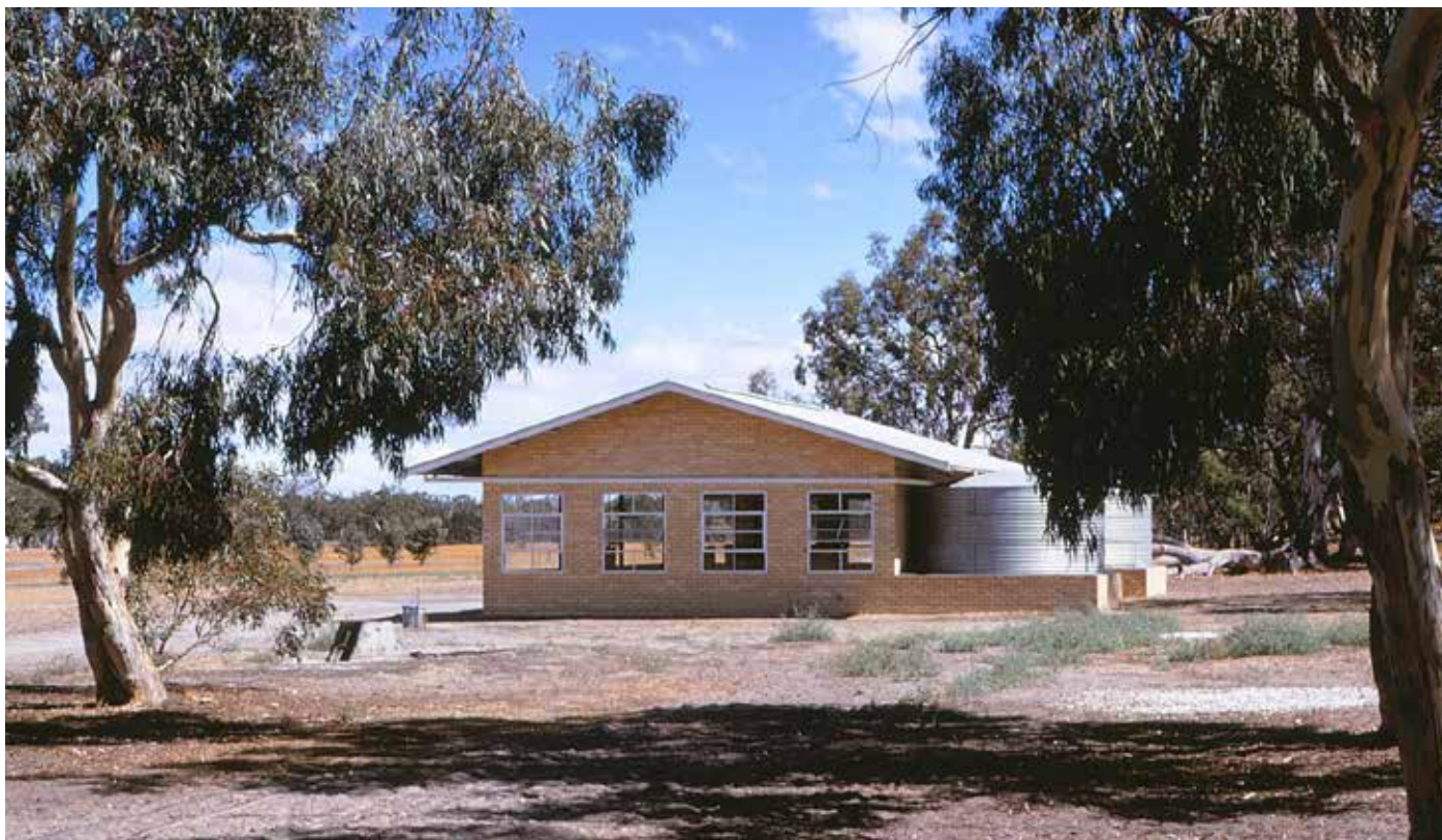
Picnic shelter erected near Wonga Hut, Wyperfeld NP, 1965-66, with a 5,000 gallon tank to collect water from the roof.
