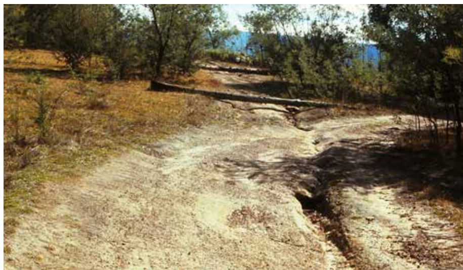
Erosion of unsealed roads was always a problem. This scene shows the erosion in Fraser NP, with the unrepaired road blocked with logs and a detour created.
