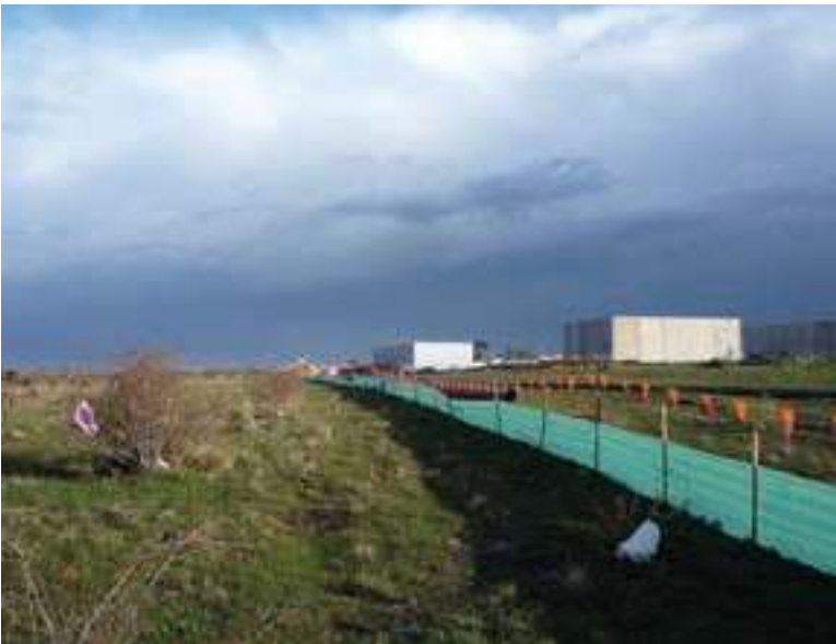
A silt fence at Craigieburn Grasslands, Campbellfield, protects grasslands during construction.
