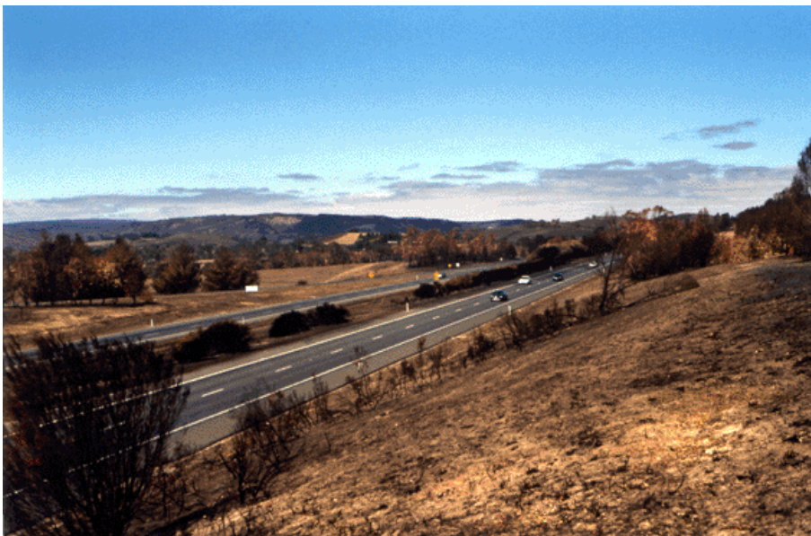
Figure 5.5 - Hume Freeway at Saunders Road overpass (26 April 2009)
